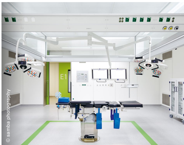
KRH Hospital Siloah Hanover, Germany
