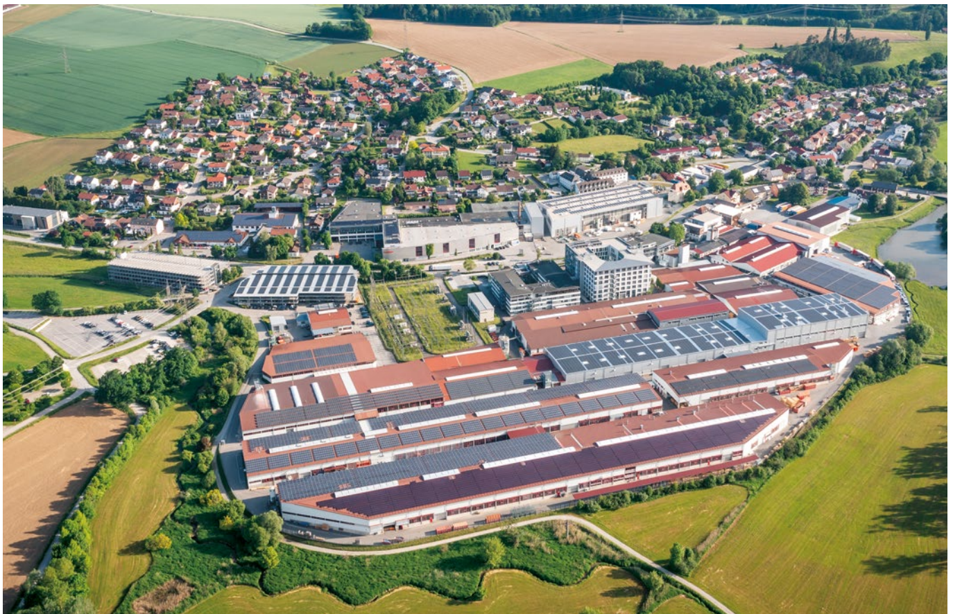
Lindner Group Headquarters Arnstorf, Germany
