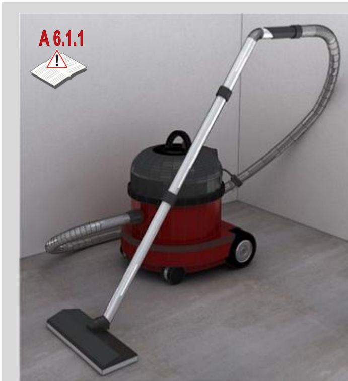
Picture 4 Cleaning of the subfloor
