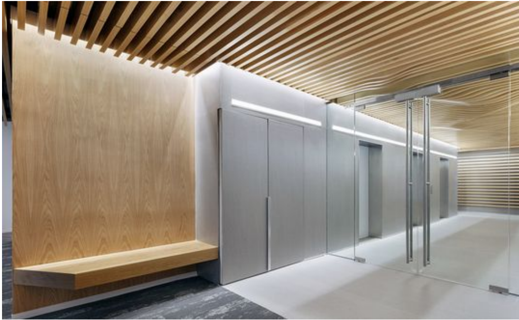
Completed Works: Custom Wood Baffle Ceiling
