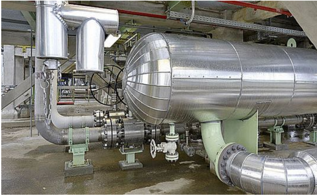
Completed Works: Industrial insulation
