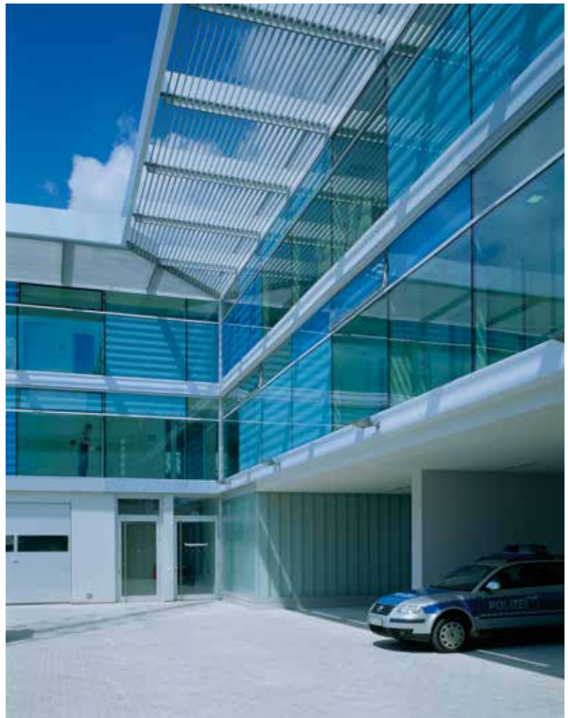
Police station, Barnim
