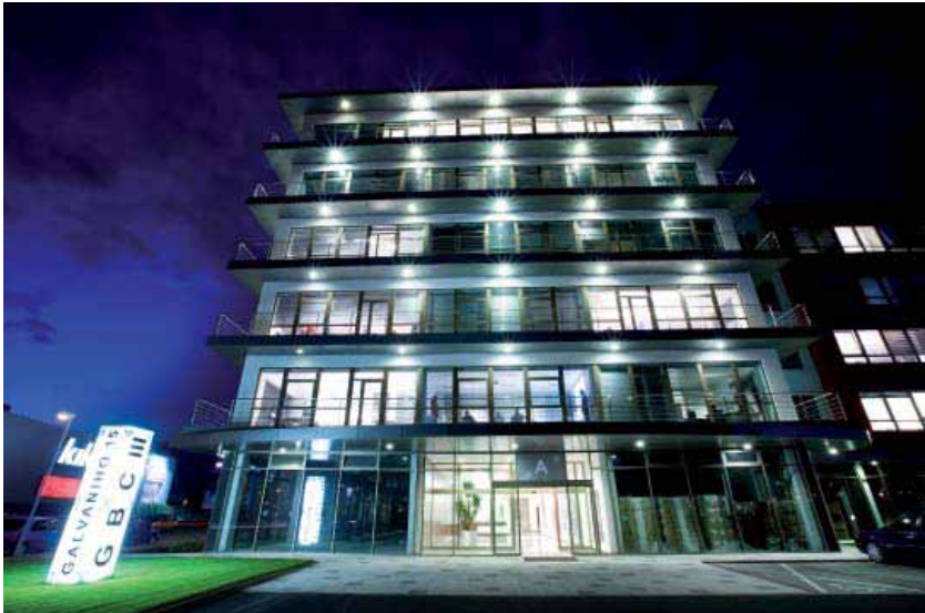
Office Building Galvaniho 3, Slovakia
