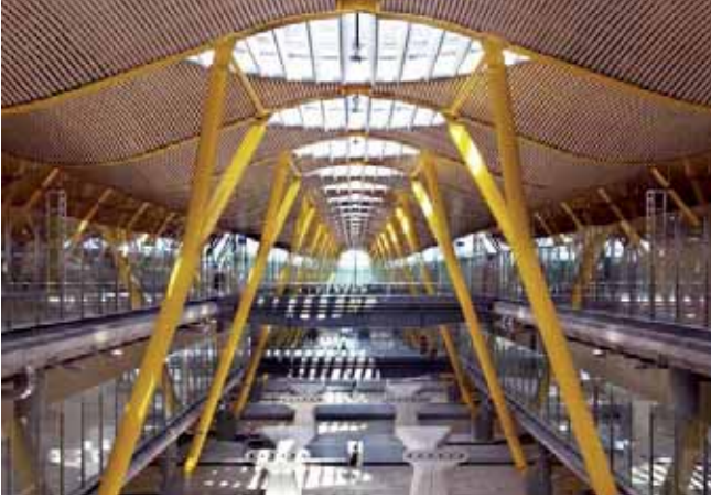
International Airport Barajas (New T4 Terminal), Madrid Architect: Rogers Stirk Harbour + Partners, Estudio Lamela Lindner handled the entire development and production as well as supplying the non-combustible bamboo ceiling.
