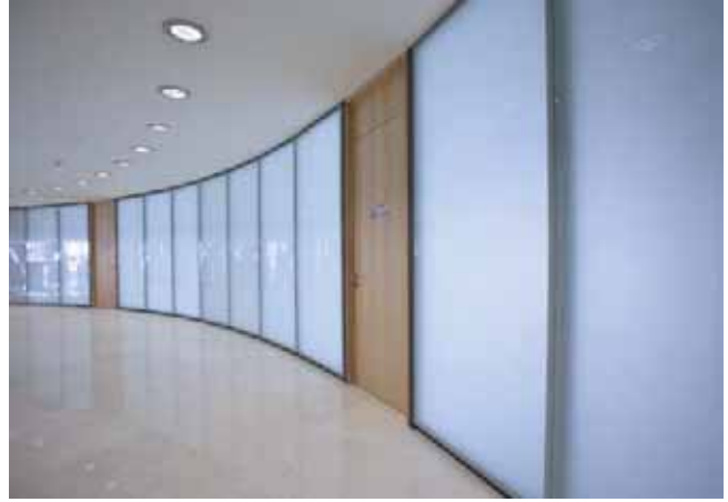
Qipco Office Tower – The Tornado, Doha Lindner supplied raised floors, glass partitions and T30 doors for this exceptional project.
