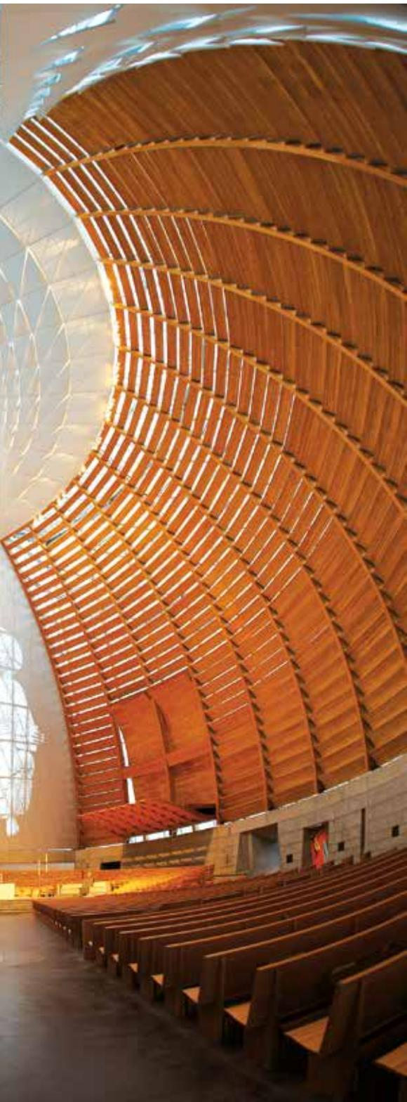
The arched wooden dome, topped by an oculus in the form of the Christian ichthys, gives an air of gracefulness to the interior. Lindner developed an earthquake-proof, Hook-On metal ceiling, consisting of large triangular plates. These were installed 36m above the ground, with a temporary level built to facilitate its installation.
