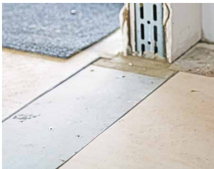
Lindner FIREport in installed condition (flat installation on adjacent floor)
