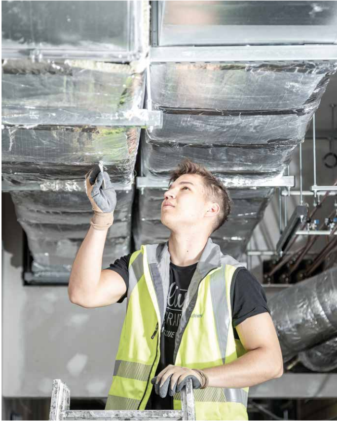
Fire protection, Deutsches Museum, Munich, Germany
