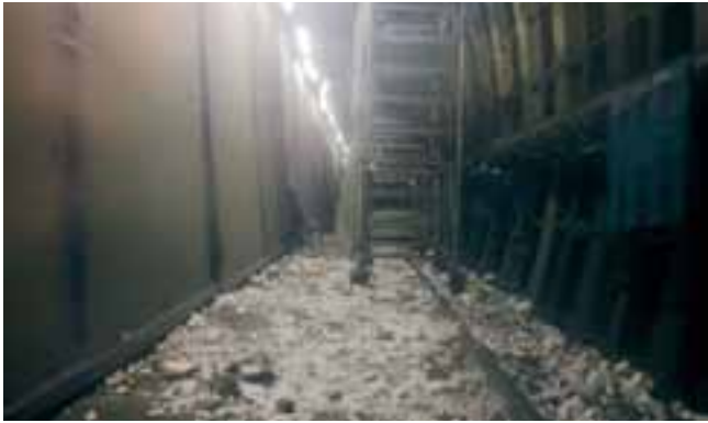
“Black Zone” - sealed off working area with spray asbestos before sandblasting.
