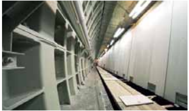
Blasted and coated steel tubing.
