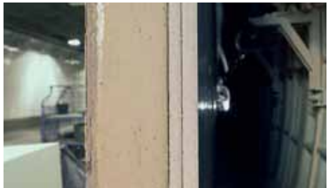
Split wall with fire protection cladding.
