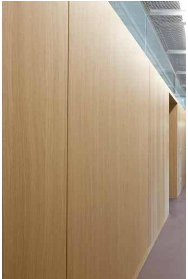
Tax office, Landshut – Timber wall cladding Lindner Free 900
