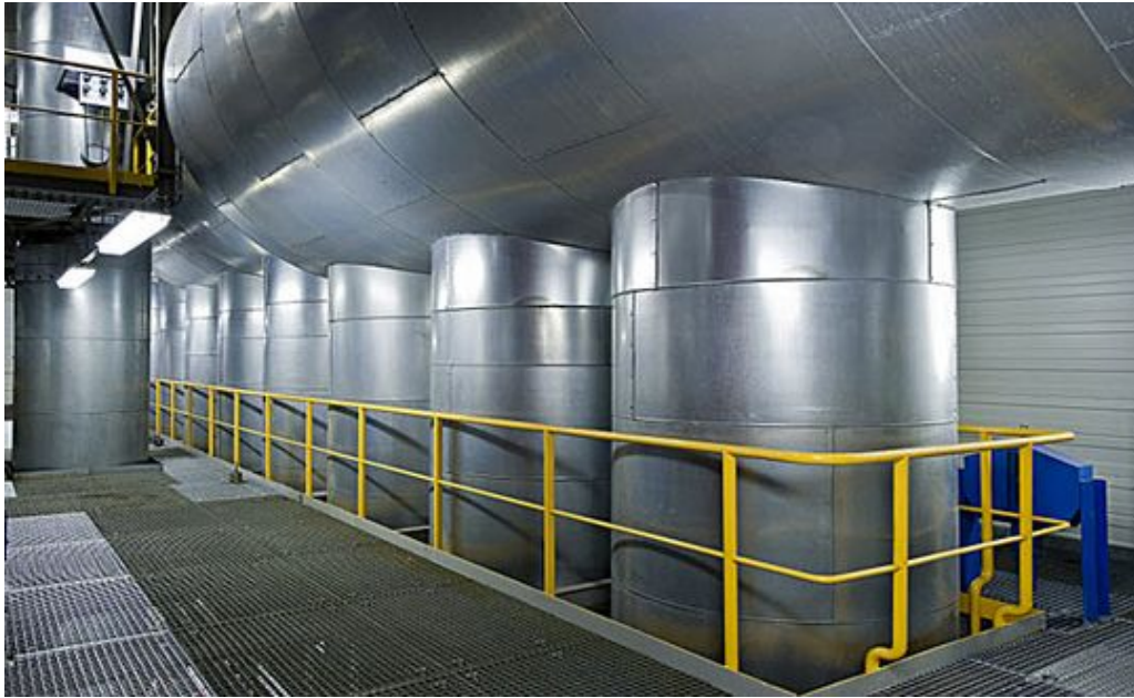
Completed Works: Insulation of power stations
