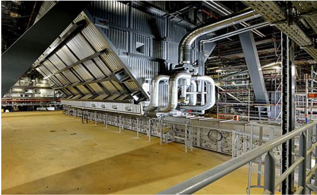
Completed Works: Insulation of power stations
